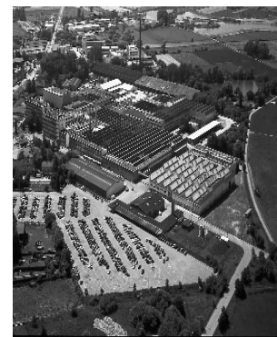
Stiebel Eltron plant in Holzminden, Germany
