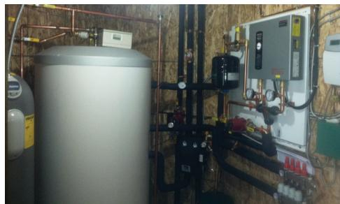
The mechanical room is compact and contains all of the solar thermal and backup equipment for the domestic water and heating system.
